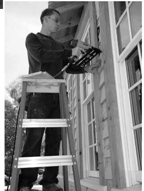
Colin Allan , of Central, a Building Construction major, has worked on the project from the beginning.
